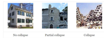
Fig. 5. Collapse check: no / partial collapse / collapse.
